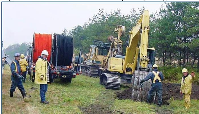
Photo 1: Underground fiber optic cable installation.
